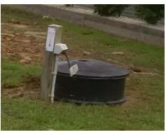
3. Remove the lid using a 3/8 hex bit, to locate the disk filter inside.
